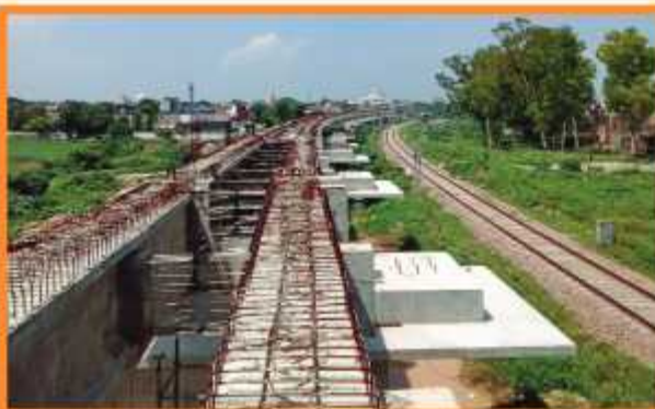
Launching of PSC Girder in Progress
