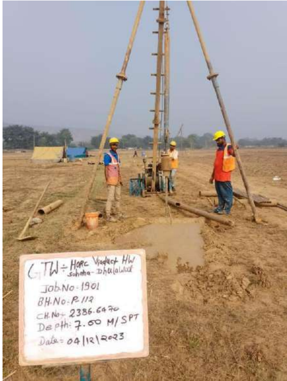
SPT at depth 7.00 m
