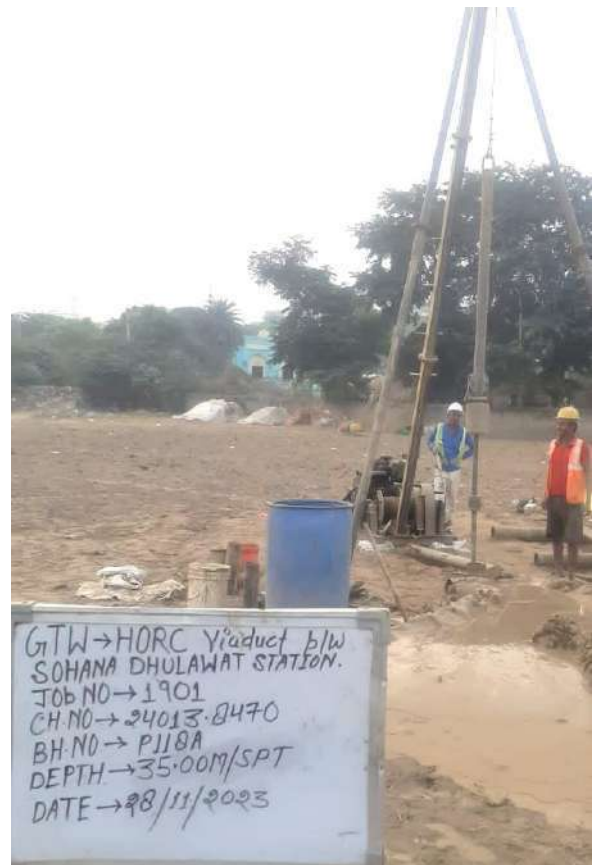
SPT at depth 35.00m
