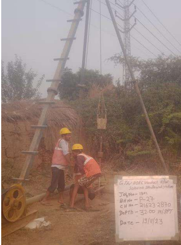
SPT at depth 32.00 m
