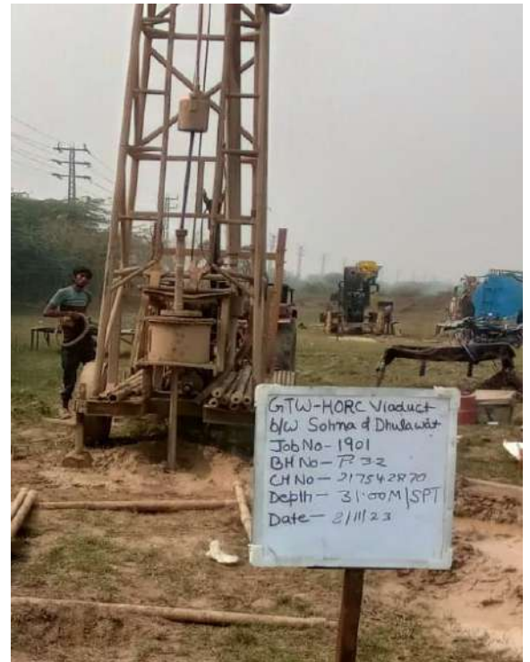
SPT at depth 31.00 m
