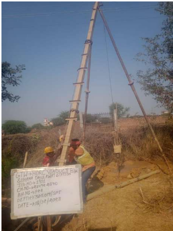
SPT at depth 30.50 m
