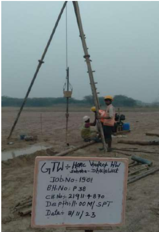
SPT at depth 11.00 m
