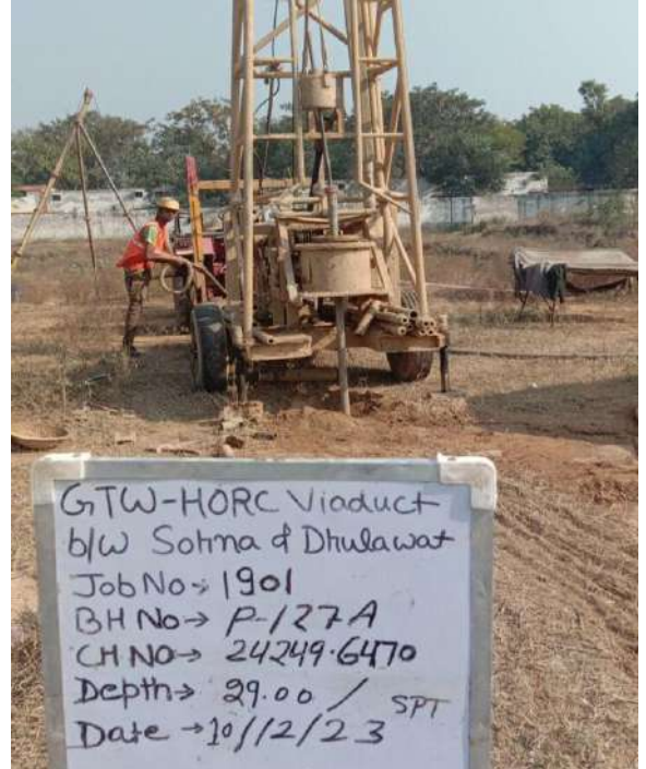
SPT at depth 29.00 m
