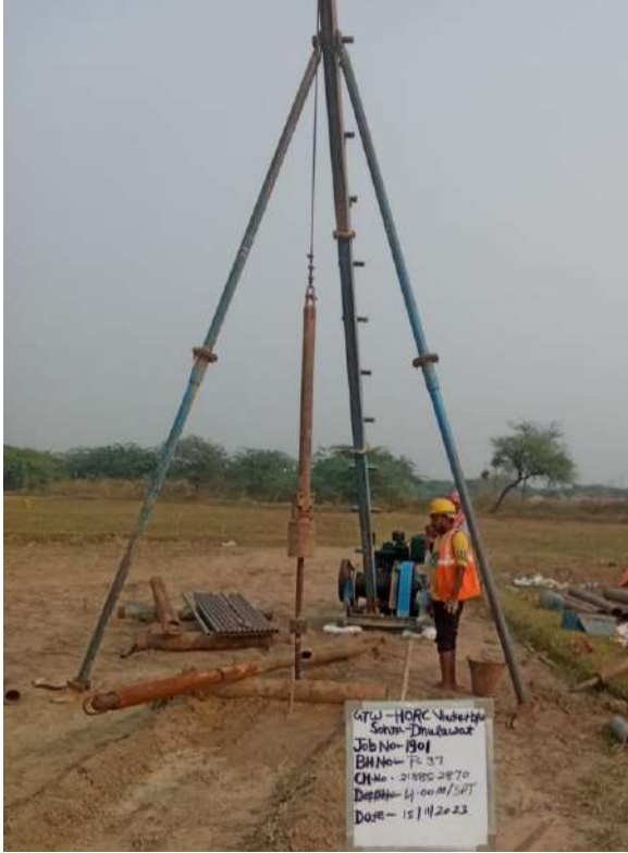
SPT at depth 4.00 m
