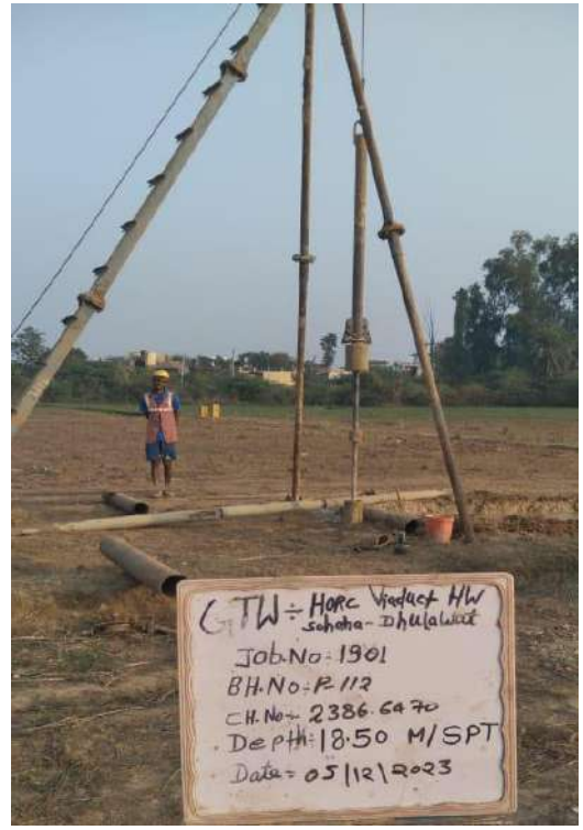
SPT at depth 18.50 m
