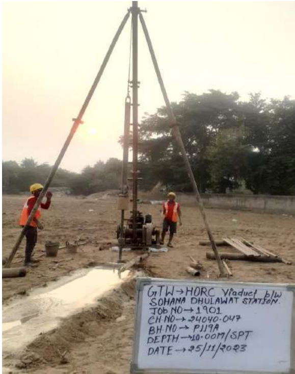
SPT at depth 10.00 m
