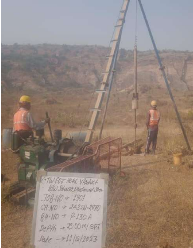
SPT at depth 29.00 m
