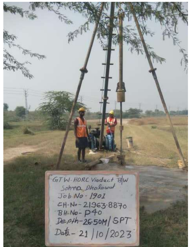
SPT at depth 26.50 m
