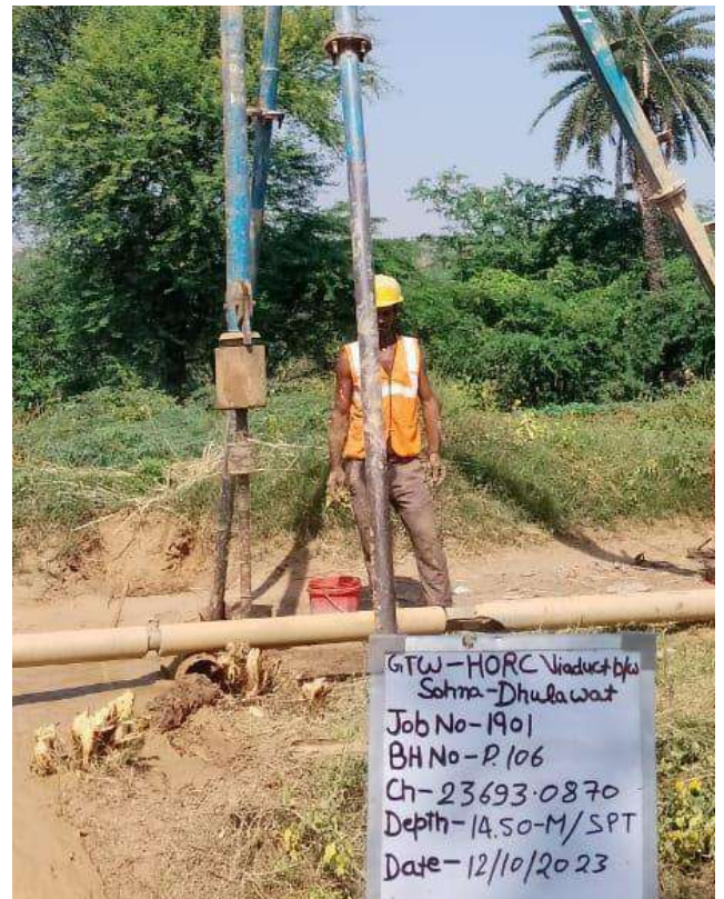
SPT at depth 14.50m
