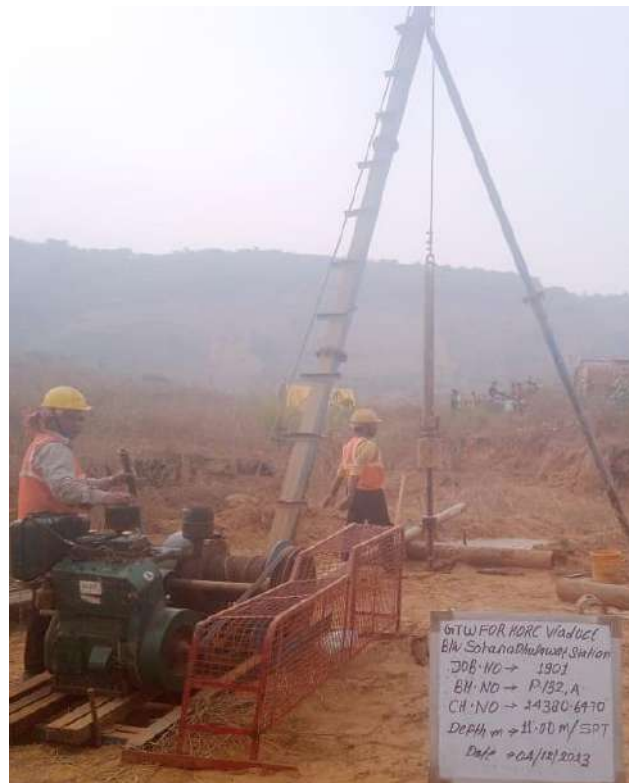
SPT at depth 11.00 m
