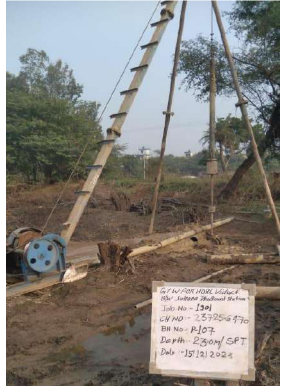
SPT at depth 23.00m
