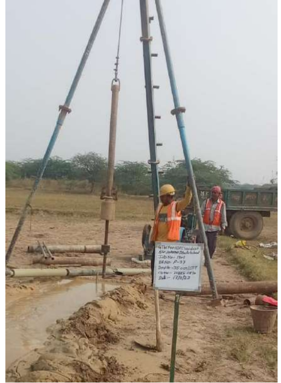
SPT at depth 35.00 m
