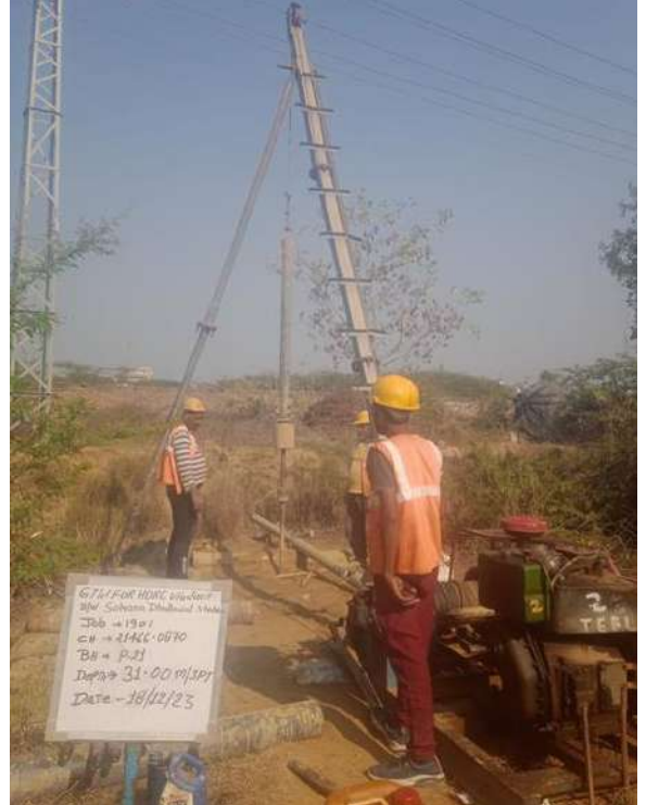
SPT at depth 31.00 m
